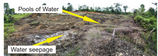
Fig. 6. View of slope from the toe (Site 2).
