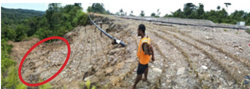
Fig. 5. View of the slope planted with Vetiver Grass (Site 2).
